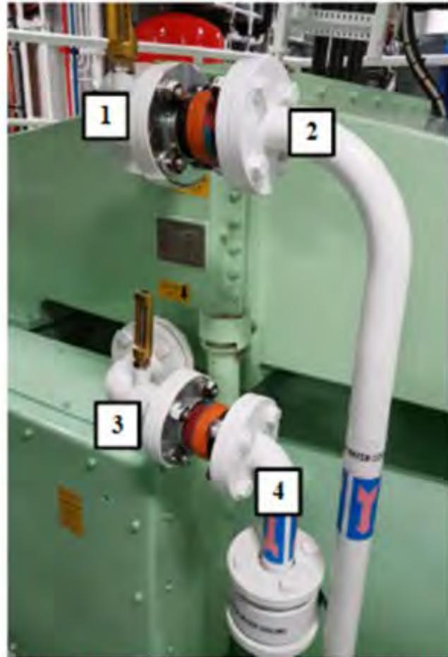
measurement positions at generator cooling pipes
